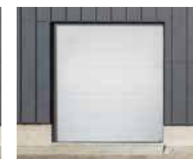
REPAIRED DOOR WITH AMARR 2747 REPLACEMENT SECTION
